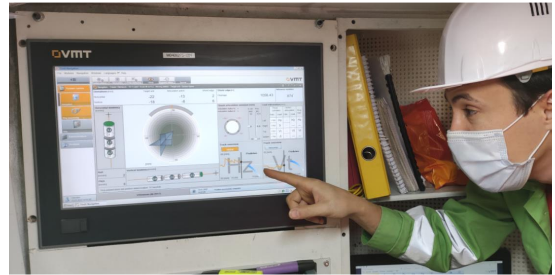
Inside the TBMs control cabin
